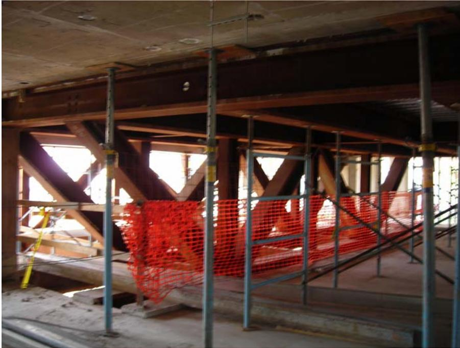
*Photo 7: Interior view of pedestrian bridge steel structure.*
